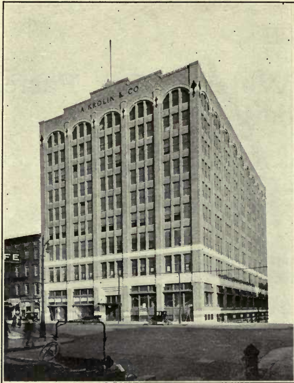
A. Krolik & Co. Building, Detroit, Michigan Albert Kahn, Architect, Ernest Wilby, Associate All concrete below grade line waterproofed with Truscon Waterproofing Paste, Concentrated . The Detroit River is directly back of the building.
